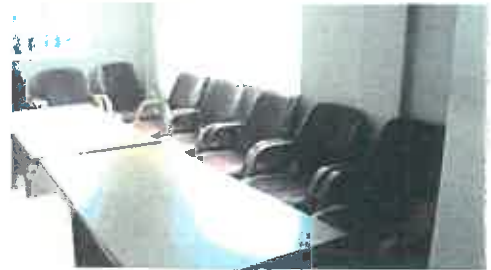
Above: Worn and torn boardroom chairs and broken table at the Bhejane traditional council
