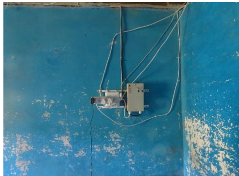
Above: Infrastructure installed in Mathunzi and a meter installed in one of the households
