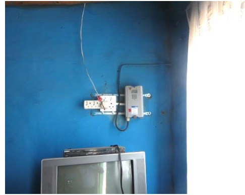
Above: Infrastructure installed in Isandlwana. Even though households have fully functional connections, households are prone to lighting strikes to a point that appliance such as televisions are damaged.
