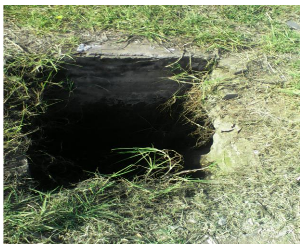
Uncovered drainage in Harding
